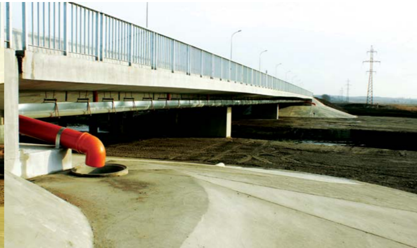
Design of a bridge over the river Zdvizh (km 51,0+845,08) REPUBLIC OF UKRAINE
