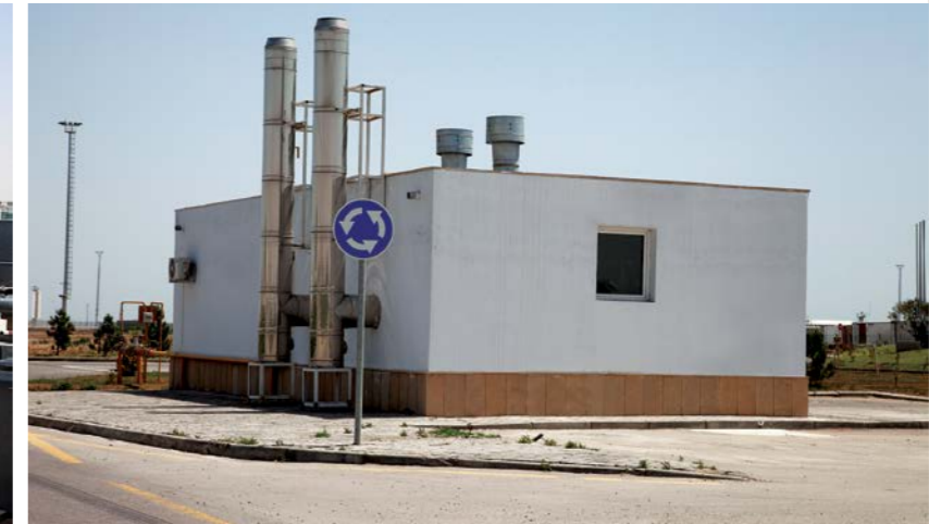
New Baku International sea trade port. Electrical Sub station Alat settlement, AZERBAIJAN REPUBLIC
